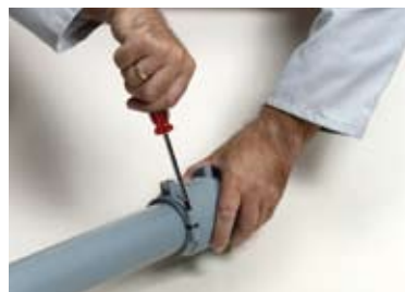
Place the pipe into the fitting and tighten the screws to fix the pipe.
