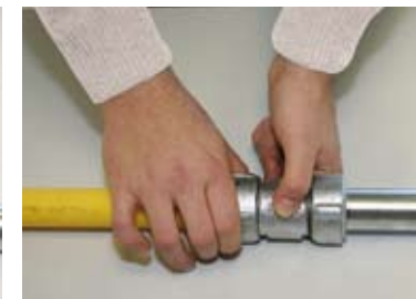
Tighten the connection by hand for a dry fit.
