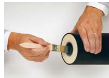
Apply the ABS Cement to the inside surface.
