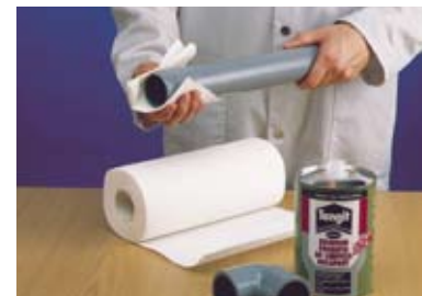
Clean the pipe and the fitting.
