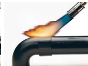
Using an open flame apply heat to the sleeve.
