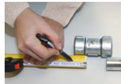
Mark the insert length of the fitting.
