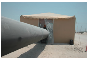
Protecting the welding zone using a tent
