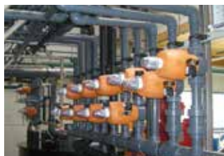
Process cooling system in PVC-U in a cable cooling station.
