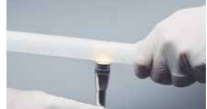
Welding quality tests on site close the extensive quality process.
