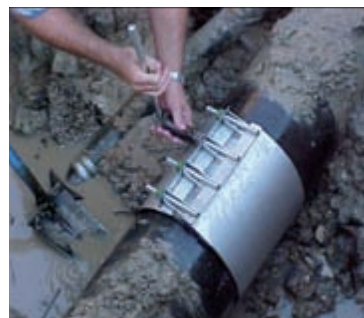
Multi/Clamp stainless steel repair clamps for emergency and under pressure repair.
