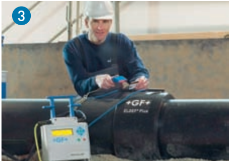
Automatic fusion data input. Easy and fast input of the necessary fusion data with the barcode reader.
