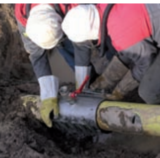
Multi/Clamp stainless steel repair clamps for emergency and under pressure repair.
