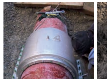
Split barrel stainless steel clamps for under pressure repair of bell & ring joint connections.
