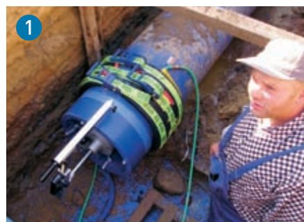
Quick and easy installation of large diameters. Active welding without preheating for diameters up to d630.
