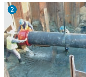
MULTI/JOINT XL fittings. Suitable to repair and maintain networks under extreme conditions and a transition for all materials.
