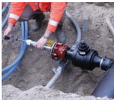
W410 drilling device for under pressure drilling through Poly-valve & ELGEF Plus branch fittings.
