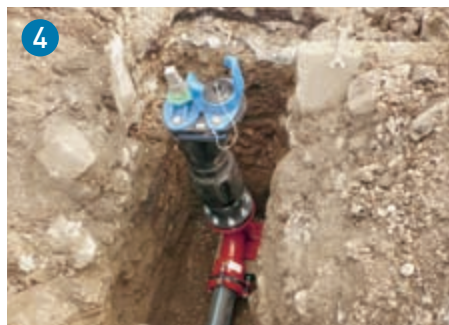
Quick and easy connections with the MULTI/JOINT duckfoot to all pipe materials and hydrants.
