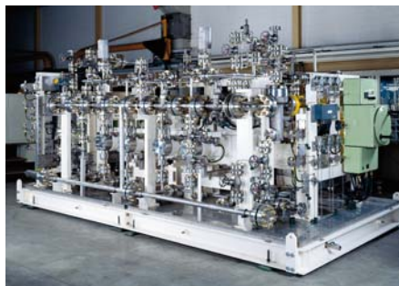
Methanol injection for offshore North Sea
