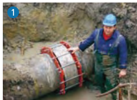
Repair of leaking joints under pressure. WAL/V leak clamps provide a dependable repair solution.
