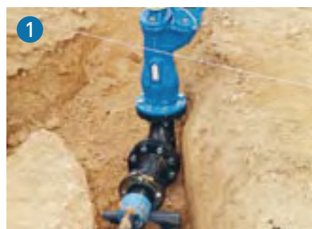
Easy connection to hydrants. Transitions between PE lines and metal hydrants are easy and safe to install.
