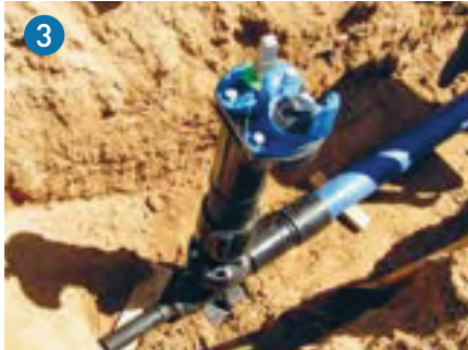
The new PE hydrant. The innovative PE hydrant can be connected using many different types of connections.
