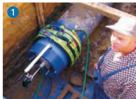
Quick and easy installation for bigger diameters. Active welding without pre-heating for diameters up to d630.
