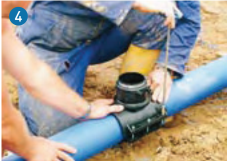
Connection to the plastic pipeline vertically or laterally. Full range of fittings which satisfy all requirements.
