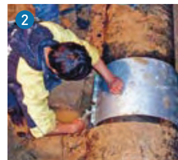
All kinds of pipe materials. For repairs up to 20 bar pressure.
