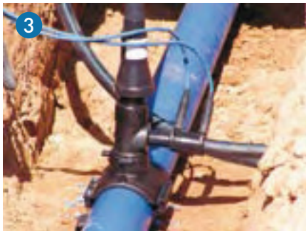
Tapping valves. Long life, choice of two tapping designs and the 360° rotatable outlet.
