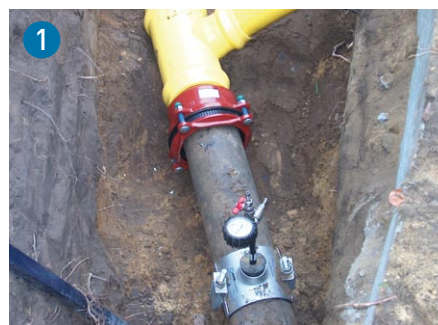
Quick gas shut-off using studded Multi/Clamp with insertable balloon.
