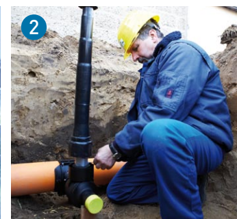
Under pressure branch connection with PE Ball Valve from ELGEF Plus with saddle and telescopic extension spindle
