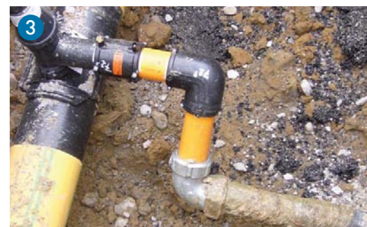
Easy and time-saving solution. Tapping saddle and Primofit combination for repair, network extension or new installation.
