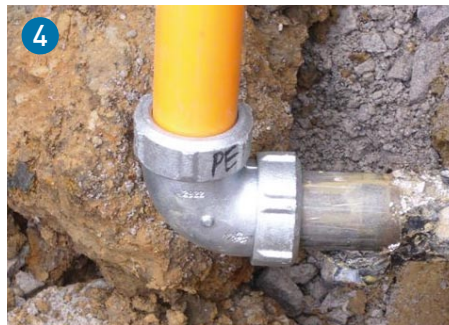
Quick restraint transition from PE100 to existing steel service lines are made with Primofit.
