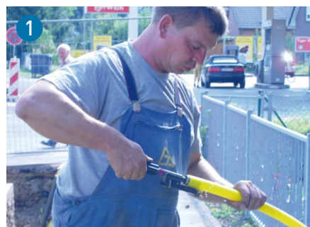
Easy preparation ensuring quality welding. Rotary scraper for correct pipe surface preparation.
