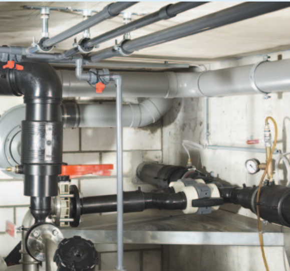
Chemical drain and waste system in CONTAIN-IT Plus or FUSEAL® (PVDF/PP).
